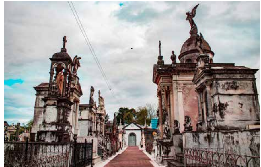
Image 1: View of the first division access.
